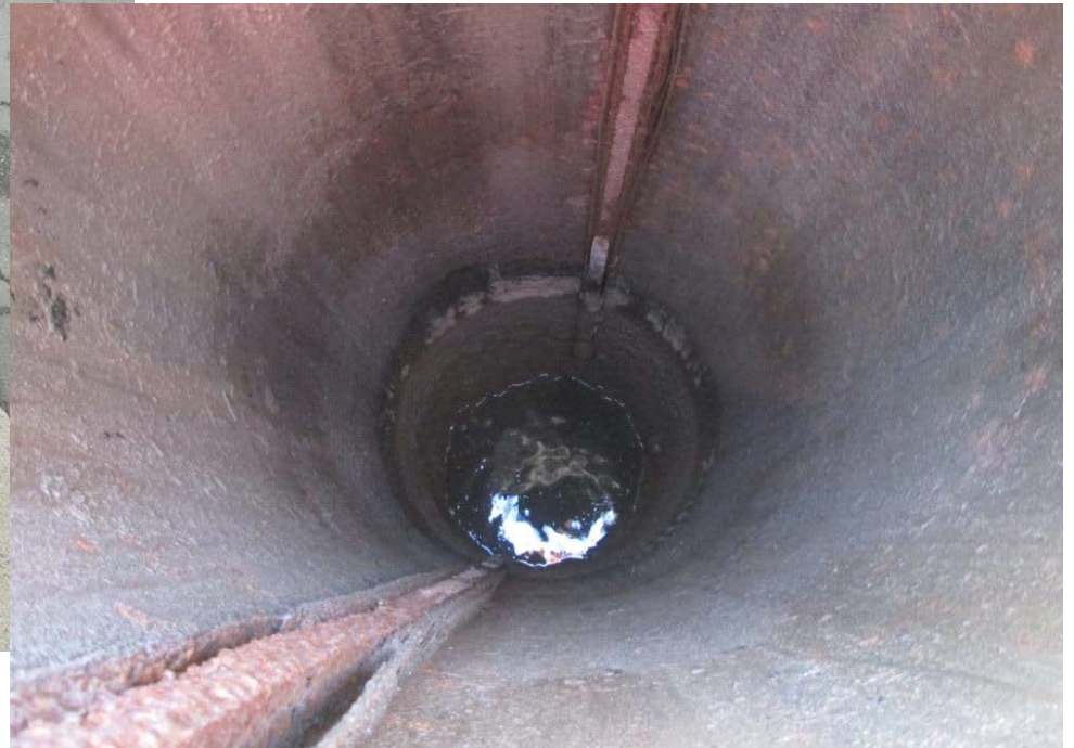
View Down Southern Manway
